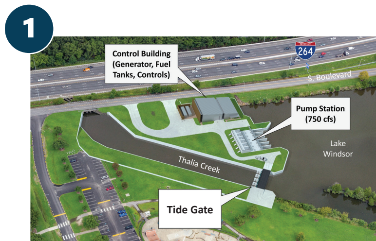
Rendering of WW Tide Gate and Pump Station
